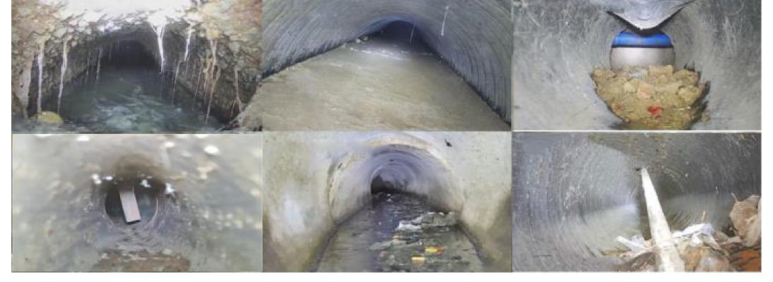
Defects in sewer pipes observed by a remote-controlled robot [4]
